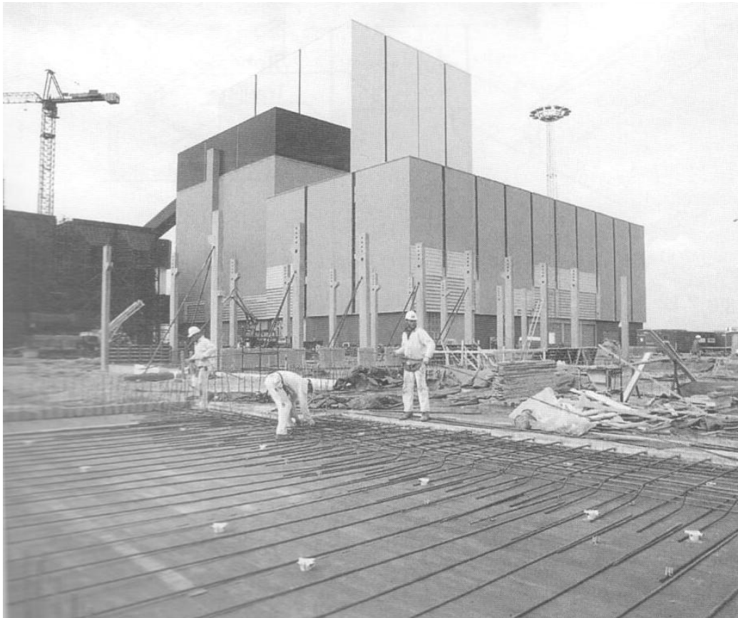
Figure 7.10: The laying down and binding of slab reinforcement
